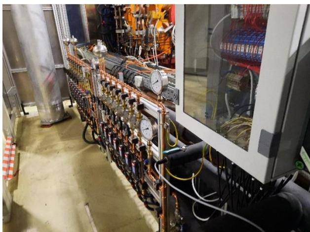
Figure 2: Water flow, pressure and temperature control of all absorber cooling circuits.
